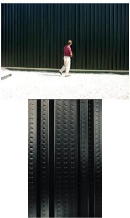
Figure 1. Transpired wall at INTEK in Aberdeen, NC. Close-up view of transpired wall shown on the right.
