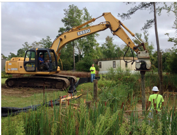
Construction workers drive the pilings that will support the Summer House in the Discovery Gardens
