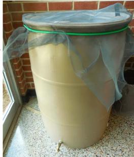
Once the barrel or cistern is full the water needs somewhere to go. It is a good idea to install an overflow pipe that allows excess water to leave the container in a controlled manner instead of spilling out the top.
