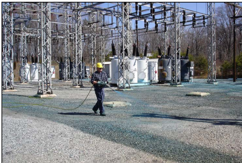
Application of pre-emergence weed control Note the use of dye to indicate coverage
