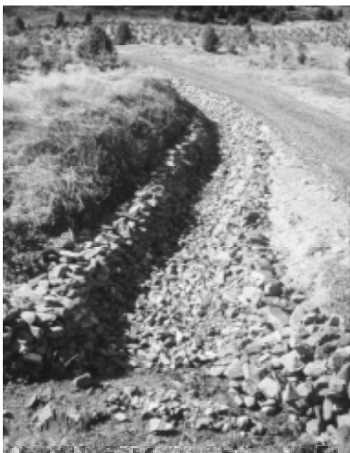
Figure 10. Proper road and drainage construction prevents erosion and reduces potential for root diseases.
