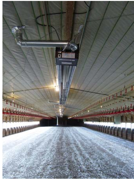
Figure 3. View of a radiant tube heater installed in a broiler house. (Courtesy: M Czarick, Univ. of Georgia)
