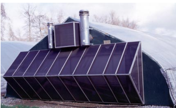
Figure 6. Insect screening is required for the prevention of Western flower thrips and other insect pests that can infest stock plants and rooting cuttings.
