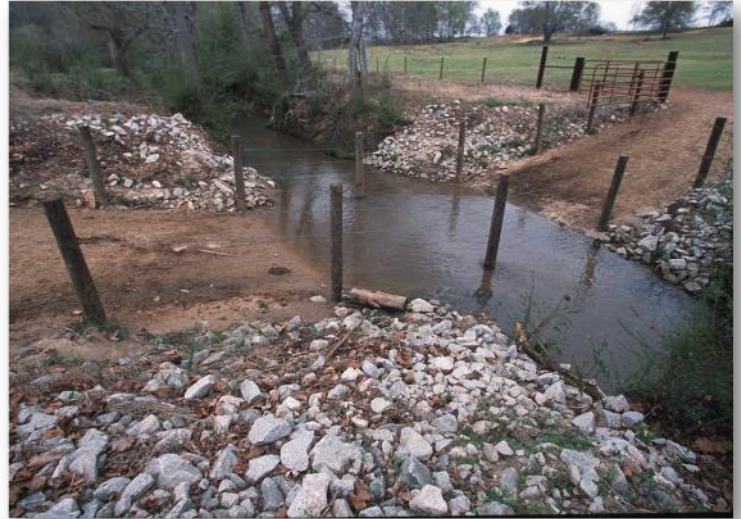
Stream crossings provide hardened, protected areas for cattle to cross
