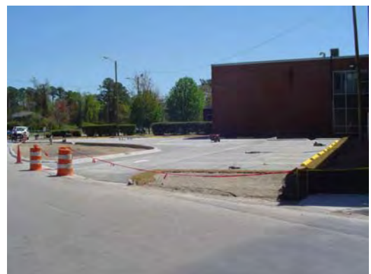
The new YMCA pervious paved lot
