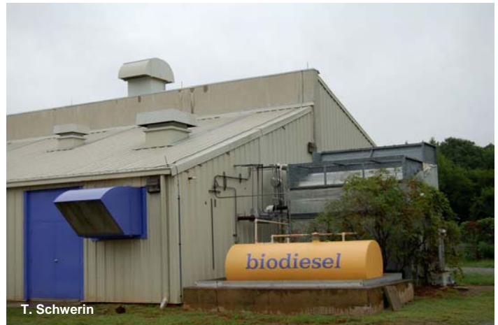
Building 3 where biodiesel is manufactured (above).
